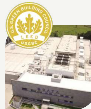
Data Center LEED GOLD
