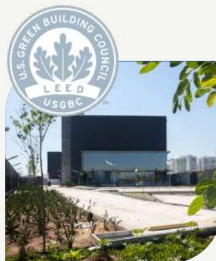
Elea Data Center LEED SILVER
